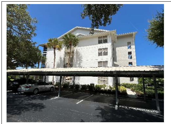
ROOF GEOMETRY – Gable/Other Roof Shape
