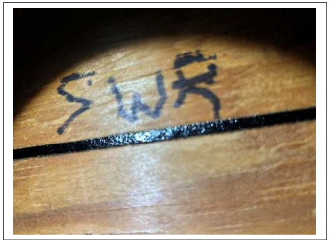
SECONDARY WATER RESISTANCE – A polymer adhesive (peel & stick) SWR barrier was installed on the entire roof deck in 2026
