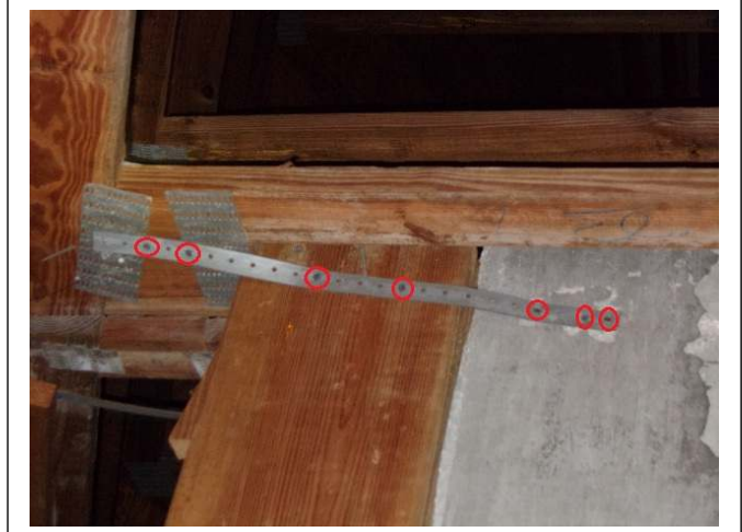
ROOF TO WALL ATTACHMENT – Metal non-wrapping straps properly secured with a minimum of 3 nails = Clips
