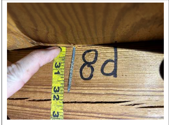
ROOF DECK ATTACHMENT – 8d ring shank nails added in 2026
