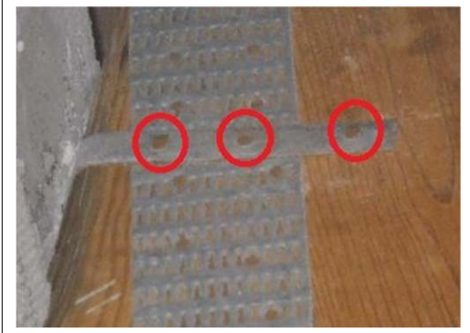
ROOF TO WALL ATTACHMENT – Metal non-wrapping straps properly secured with a minimum of 3 nails = Clips
